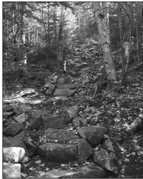
New MCC stone staircases on the Pond Link Trail
